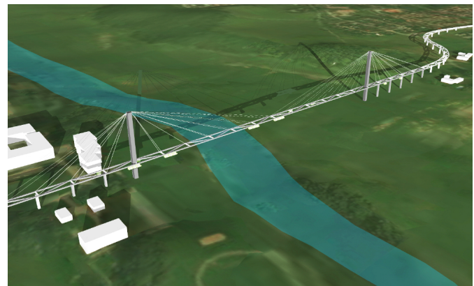
Fig. 2.1b Cable-stayed GTS bridge over River Fyris (AyCrete/Joakim Gustafsson)
